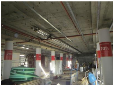
Construction on the 2nd basement level
