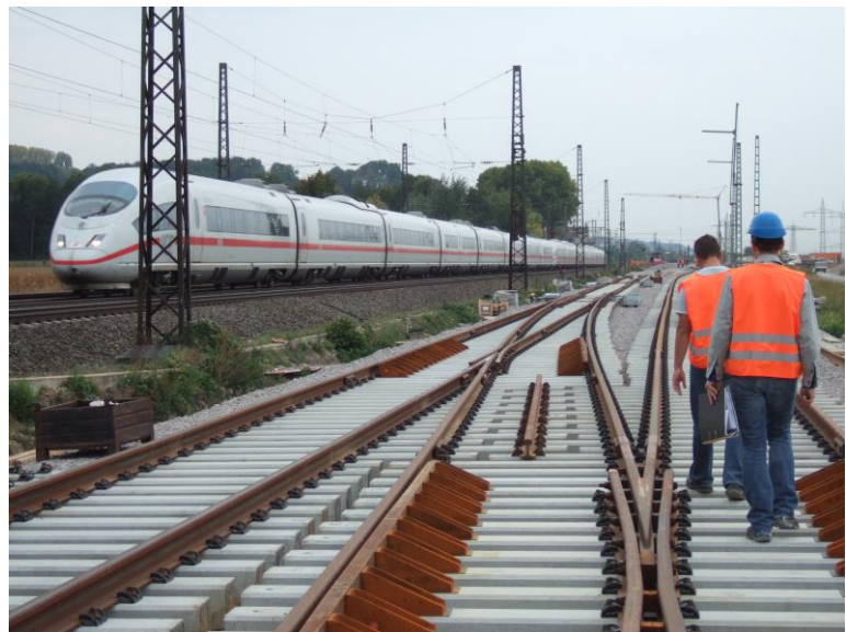
Upgrading of the Katzenberg Tunnel connection to the old Rhine Valley Railway to 4 tracks during railway operation
