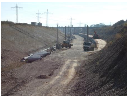
Deep connection cuts
