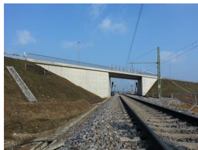
Münchner Strasse road crossing, km 71.998
