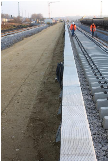
New station, Baar-Ebenhausen
