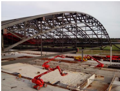
Construction of the roof structure
