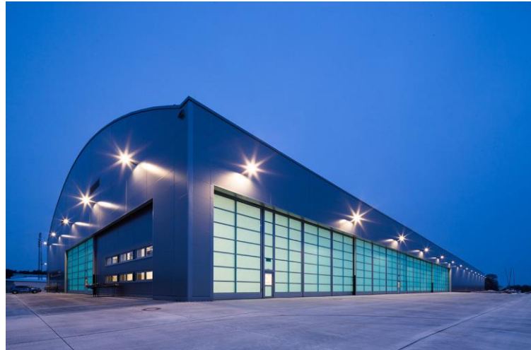
New maintenance hangar
